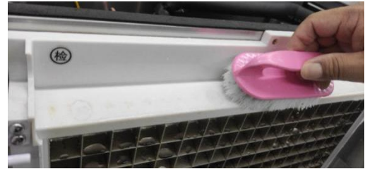
Brush the plastic parts around the evaporator
